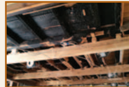
"The most difficult part of the renovation," says Borkowski, "was dealing with the deterioration of the existing structure, substandard construction practices during earlier renovations, and the structural damage caused by two or three different fires that had taken place."
